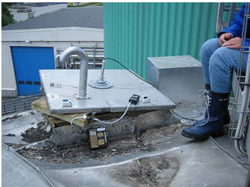
Figure 9: Picture of sampling inside the buffer tank
