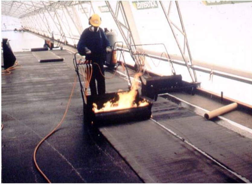
Figure 8. Torch-welding of bitumen sheet
