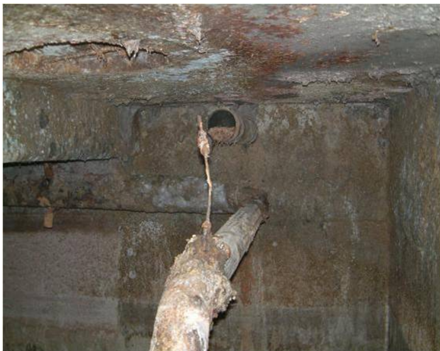
Figure 1. Corrosion damage on tank in biogas plant [Boubitsas 2010]
