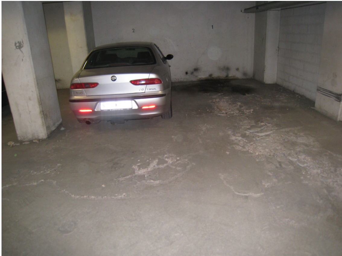
Figure 2. Concrete damage in a garage
